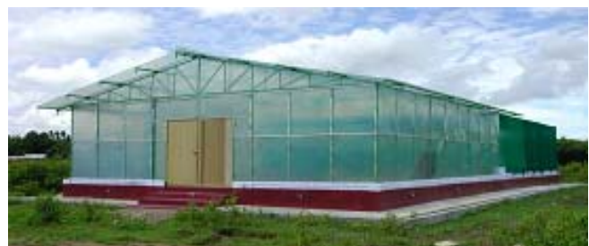
Shade cum poly house constructed under MoEF funded project for development of botanical garden at RFRI
