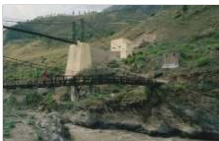
Project Site-Tapovan Vishnugad Hydroelectric project
